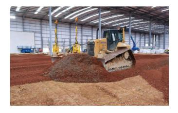
Our Laser Levelling system can prepare large areas of stone/sand blinding very efficiently and accurately, up to 3200m<sup>2</sup> per day. We are able to level all types of aggregates leaving no 'track' marks in the stone and without damaging pile caps or penetrating the sand blinding which we are levelling thus providing a smooth working surface for the customer.
